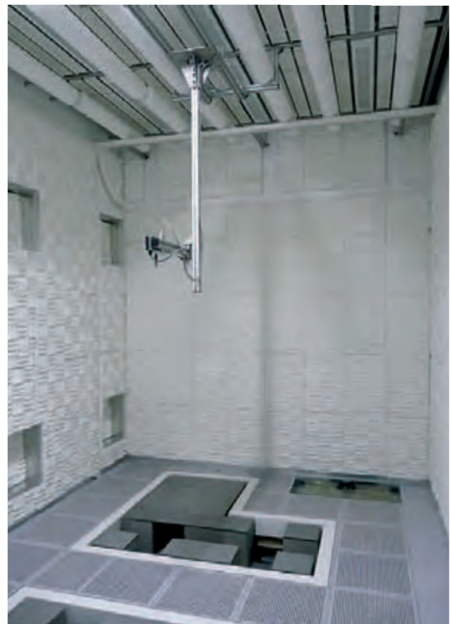
Experimentation room with 4.2 m clear room height and acoustic insulation materials (supplied and installed by Bilz).
